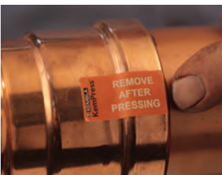
Pressed fitting - indents on the fitting.
