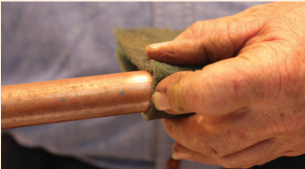
3. For existing copper tube, clean the end with emery paper or a soft scourer.
