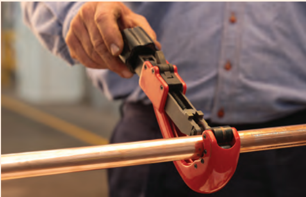
1. Cut copper tube to length using a pipe cutter.
