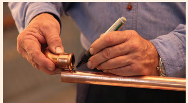
4. Mark the insertion depth by lining up the fitting side by side with the tube and mark the tube. When the fitting is inserted onto the tube the outer edge of the fitting must line up with the marking. For correct insertion depths see column e of the Fittings Space Requirements table, page 20.
