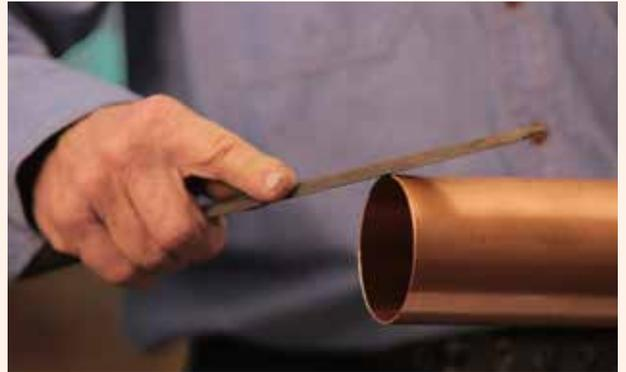
**2.** Carefully deburr and wipe clean the end of the tube internally and externally to minimise turbulence and pressure loss according to AS3500 and avoid damaging the O-ring.
