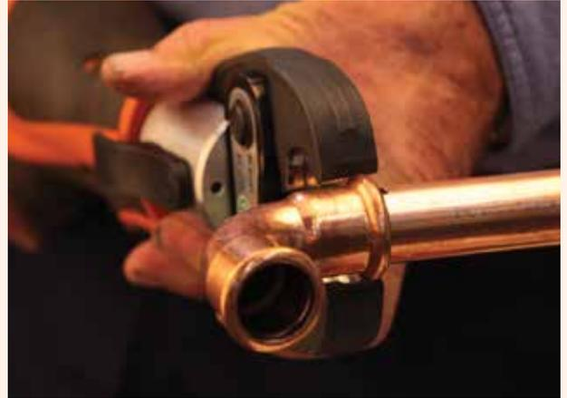
**7.** Check the fitting outer edge still lines up with the marking. Open the pressing jaw and close it around the fitting so the raised bump in the fitting rests inside the groove of the pressing jaw.
