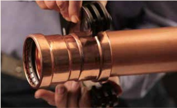
**7.** Open the collar and place it around the fitting, such that the bump on the fitting is rested into the groove of the pressing collar. Close the press collar ensuring it fits square with the fitting and check the insertion depth mark still lines up with the outer edge of the fitting.
