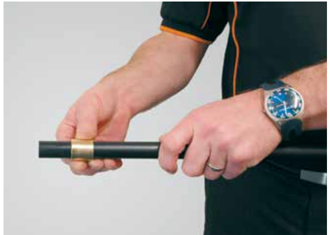
2. Slide on brass sleeve with chamber facing toward fitting
