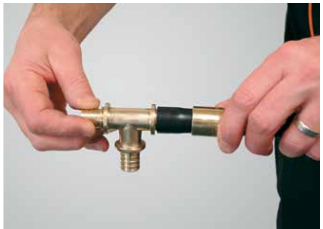
6. Fully insert fitting into tube
