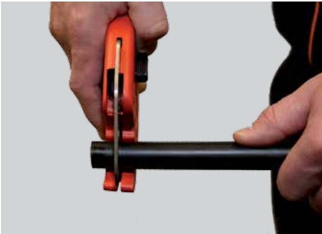
1. Cut pipe at right angle.
