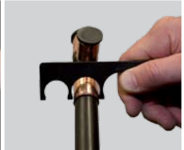
6. Test with Kembla Press gauge
