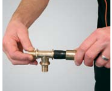
6. Fully insert fitting into tube
